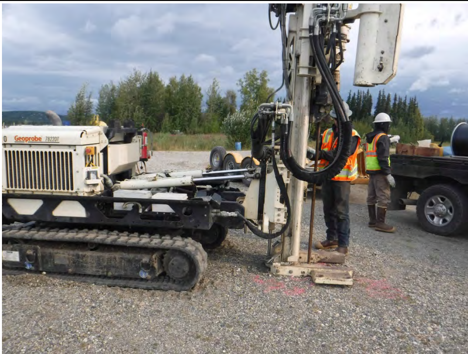
Description: Temporary monitoring well TW101 location during installation.
